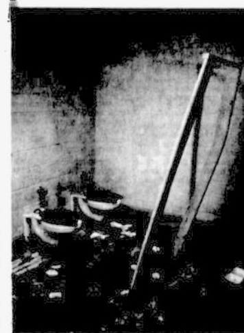
Toilet stalls have been ripped down; toilets are backed up and rubble covers restroom floors at Zumwalt Park on Fern Ridge.
