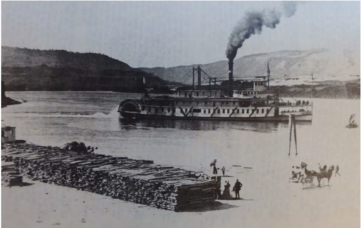
Fig. B3.5. Photograph by H.G. Miller from about 1915 of the river steamboat "Bailey Gatzert" in the vicinity of The Dalles. The "Bailey Gatzert" made regular runs between Portland and The Dalles from 1900 to 1917. The Cascade Locks, completed in 1896, made it possible for vessels to travel up the Columbia River as far as The Dalles without portaging. Note wood stacked on the beach awaiting shipment. Pieces are relatively short and have been split rather than cut, suggesting they are intended as firewood. It is impossible to say from this photograph whether the wood is pine or oak. 39
