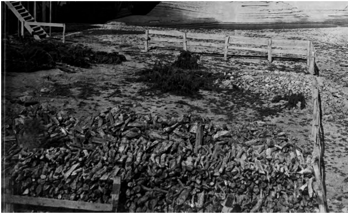
Fig. B3.1a. Detail from lower left of Fig. B3.1 showing wood pile below steamboat wharf. The wood appears to be oak, comprising mostly smaller diameter limbs.
