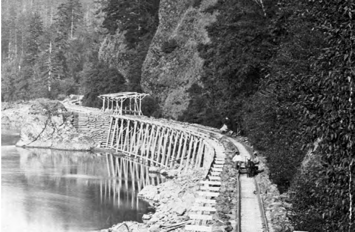
The tramway constructed by Joseph Ruckels and Harrison Olmstead at Tooth Rock on the south shore of the Cascades. This so-called railroad consisted of a simple wagon drawn by a mule. The tracks were wooden stringers with a strip of metal laid over the top. The original Cascades portage railway, constructed by Francis Chenoweth on the northern shore of the river, utilized similar technology. [Oregon Historical Society, "Carleton E. Watkins photographs, 1861-1885"; Org. Lot 93; OrHi 21575]
